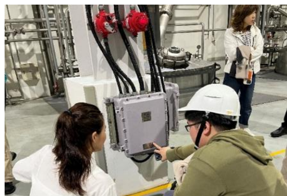
03.2025 Engineer Kai-Hong You (R) conducted explosion-proof electrical assistance at a chemical materials plant.
