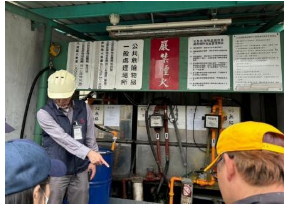
02.2025 Senior Technical Manager Ching-Fong Lin (L) conducted explosion-proof electrical assistance at an automotive parts factory.
