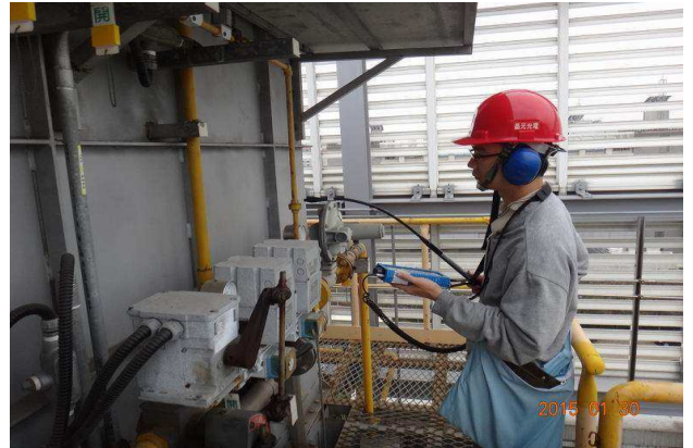
05.2014 Ultrasound testing, Engineer Di-Lung Tsen
