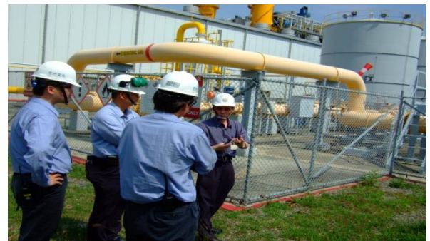
05.2015 Explosion-free electric zoning for a nature gas power plant, Senior Engineer Qing-Feng Lin (R1).
