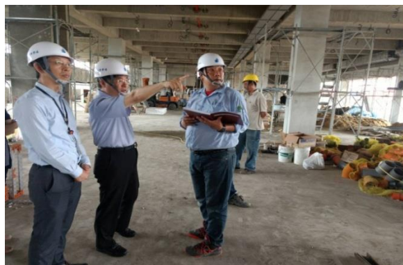
07.2017 Hi-tech facility fire protection assessment- VP Dr. Cheng-Chang Huang (C).
